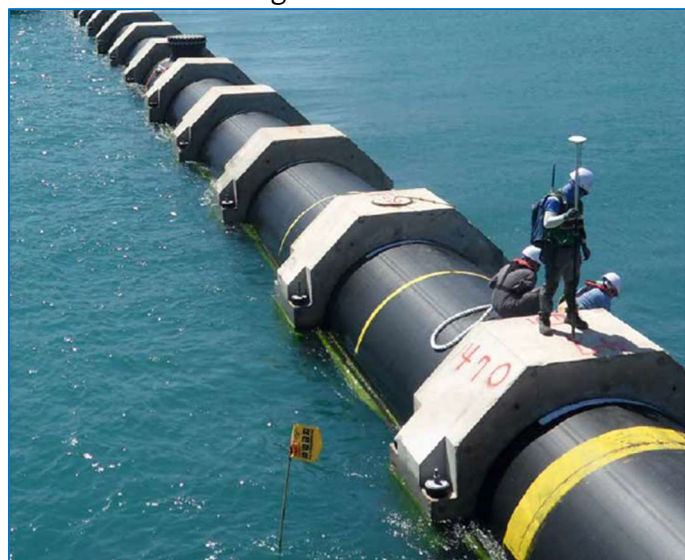
Octagonal Anchor Blocks
