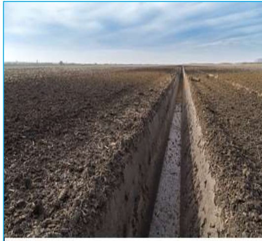
Open trench method
