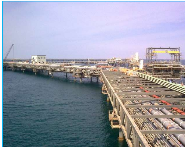
Laying of trestle
