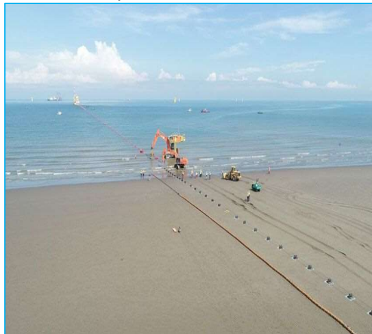
Alignment of pipeline
