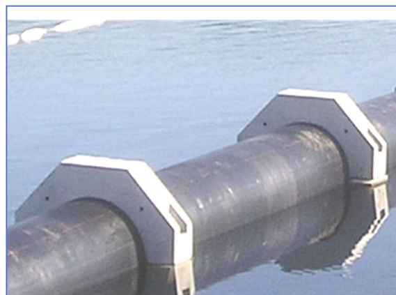
Concrete Blocks with HDPE Pipe
