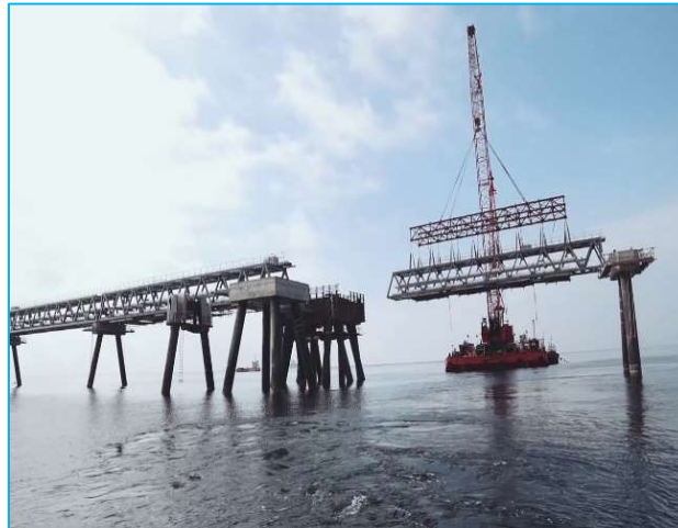
Construction of trestle
