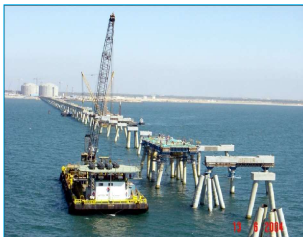
Alignment of trestle
