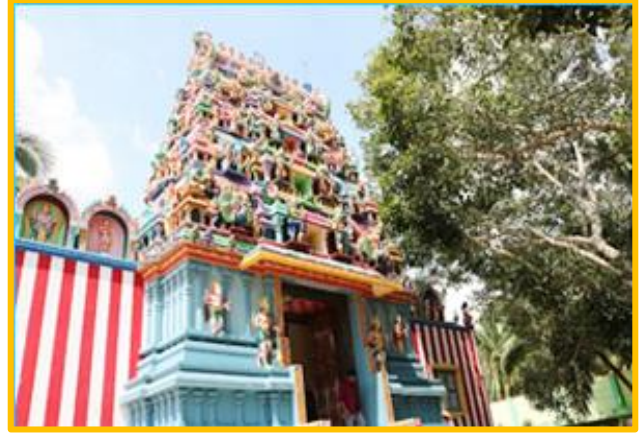
Entrance after construction of Rajagopuram
