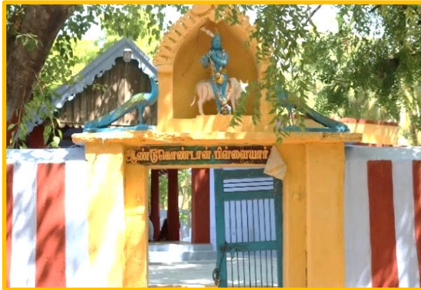
Entrance before renovation of Rajagopuram
