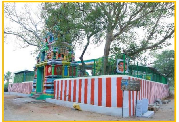
Compound wall at present
