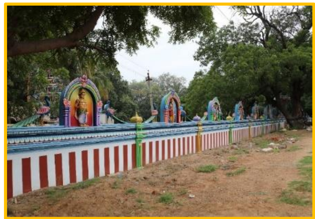
After the completion of compound wall
