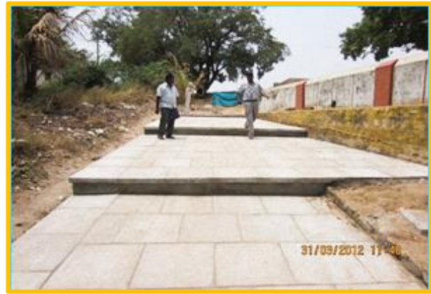
After completion of stone pavement
