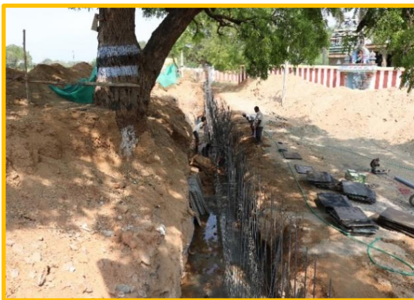
Before the construction of Compound wall
