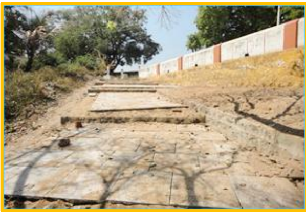
Construction of stone pavement in progress
