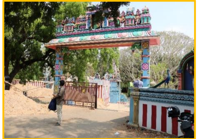
Entrance Arch with compound wall
