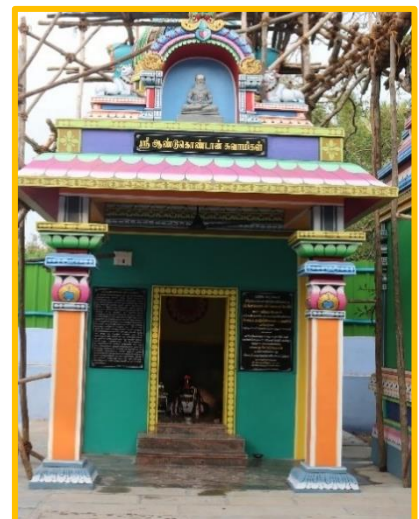
Shri Andukondan Swamigal Sannadhi after renovation
